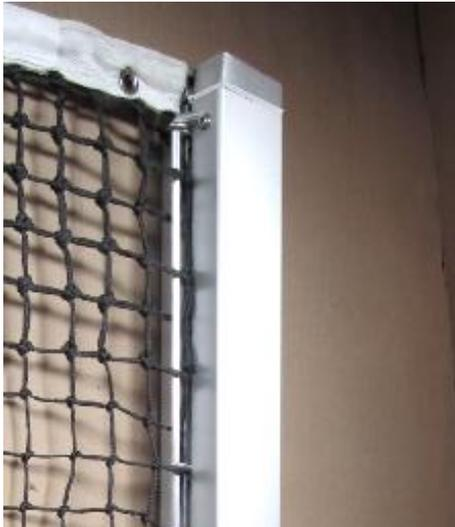
Afterwards also push the net holding rod through the net hooks and pull the net evenly over the rod. If there are additional fixing ropes at the net pull and fix them around the upright. Then the net can be tensioned as requested.
