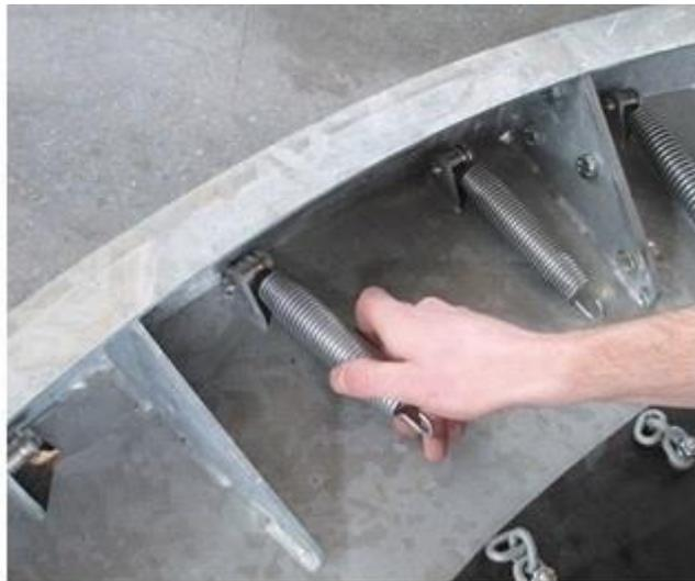
**Matting membrane with tensioning belt on chain link and spring bushing Fasten. Start with the assembly of the spring.**
